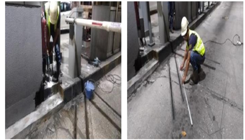
4 Replacement of Loop Coil for Lane at SILK
