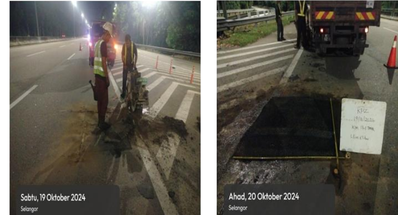
Pavement Spot Repair at SILK
