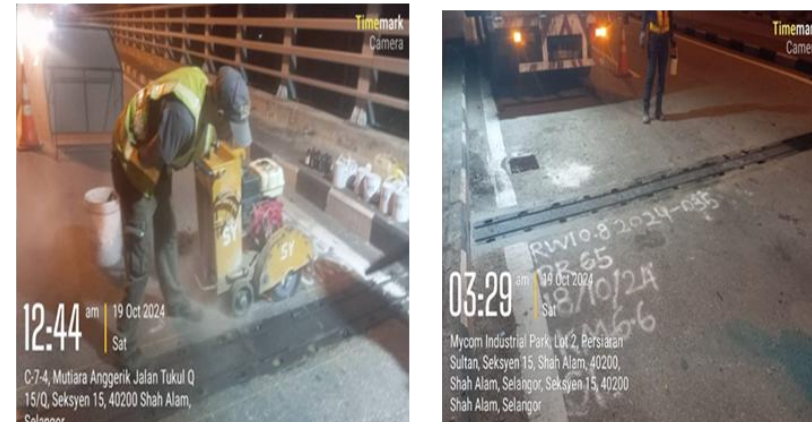
Pavement Spot Repair at SILK
