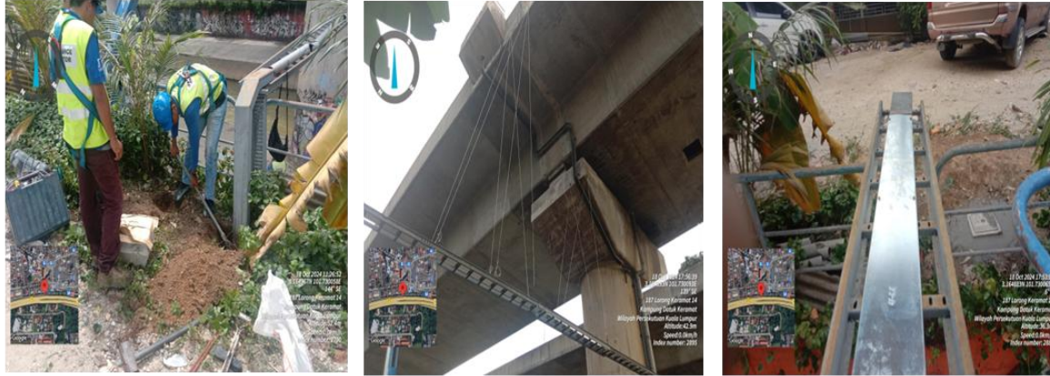
3 Lay Power Cable For CCTV And VMS at SILK
