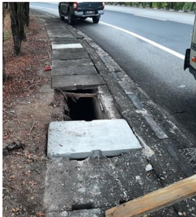
Replacement of Damaged Pre-cast Concrete Slab at LKSA
