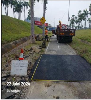
Replacement of Damaged Pre-cast Concrete Slab at LKSA
