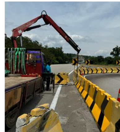
Installation of New Concrete NJB at SILK
