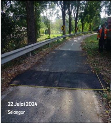
Replacement of Damaged Pre-cast Concrete Slab at LKSA
