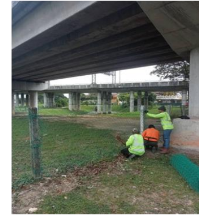
4 Installation of ROW Fencing at LKSA
