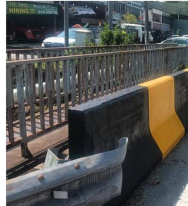
Installation of New Concrete NJB at SILK
