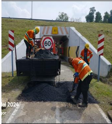
Replacement of Damaged Pre-cast Concrete Slab at LKSA
