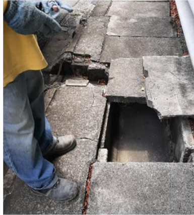
Replacement of Damaged Pre-cast Concrete Slab at LKSA
