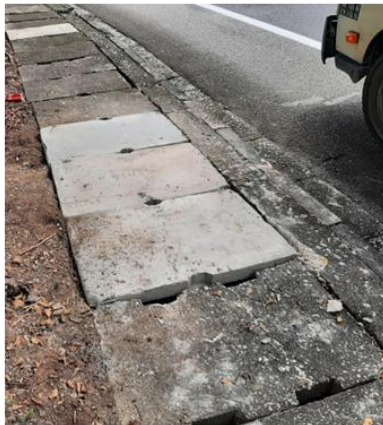
Replacement of Damaged Pre-cast Concrete Slab at LKSA
