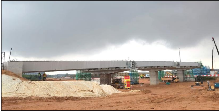
Launching of U14 Beam at Zone B
