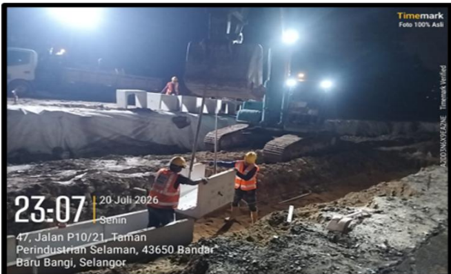
Installation of U-Drain (600mm x 600mm) at Stage 5A-2 (Ramp 2G) from CH175 to CH300
