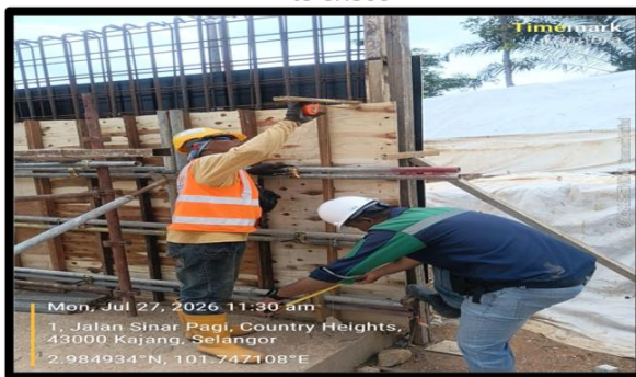
Installation of formwork prior to concreting the RC Wall construction at Stage 5A-1 (Ramp 2F)
