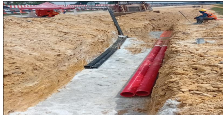
Installation of 2-ways PN10 & PVC Pipe for TCSS & TNB Relocation Work
