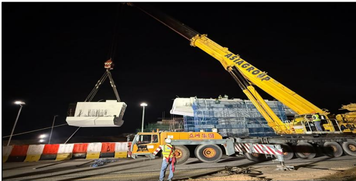
Launching of Segment 3 of Crosshead for Pier 3 (Median)
