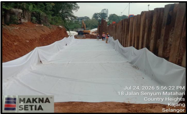
Filling work for Remove & Replace (R&R) Widening Work at Stage 5A-1 (Ramp 2F)
