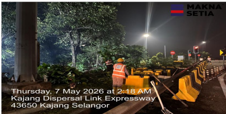
Trees cutting works & Concrete Barrier Arrangement at Stage 5A-1
