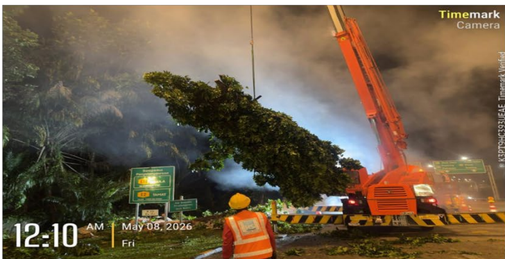
Tree cutting works at Stage 5A-1 (Ramp 2F)
