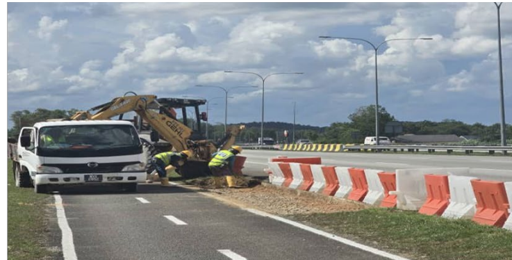
Preparation to Activate TMP Stage 1 (Motorcycle Lane Closure)
