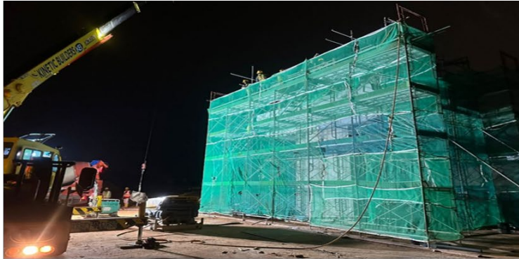
Concreting Work for Segment 1 at Pier 6 (Infill)
