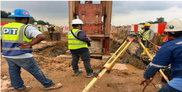
Sonic Logging Test at Pier 3-3
