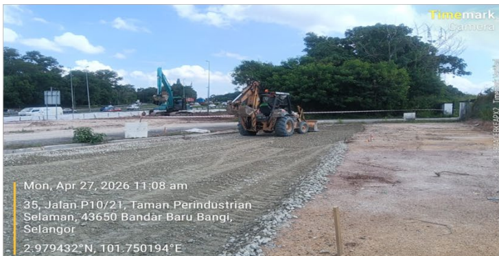
Crusher run lay for slip road graveyard area (Stage 5A-2 – Ramp 2G)
