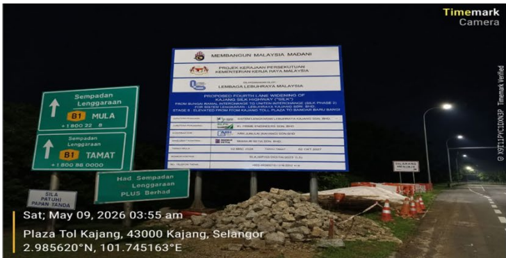
Installation of project signboard at CH. 0
