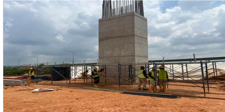
Platform Installation Work for the Launching of Precast Segmental Crosshead
