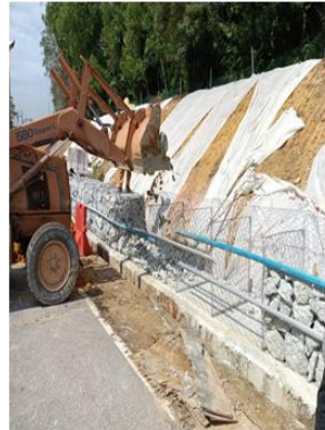
Rehabilitation Works for Slope
