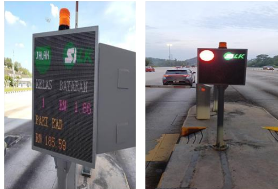
Replacement of Full Color LED Toll Fare Indicator
