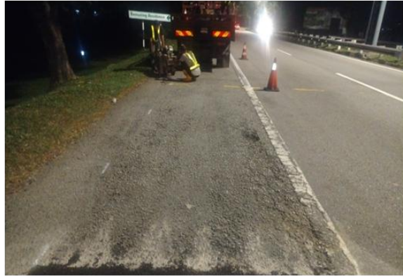
Pothole Repair
