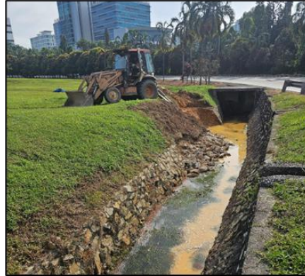
Rehabilitation Works for Drainage
