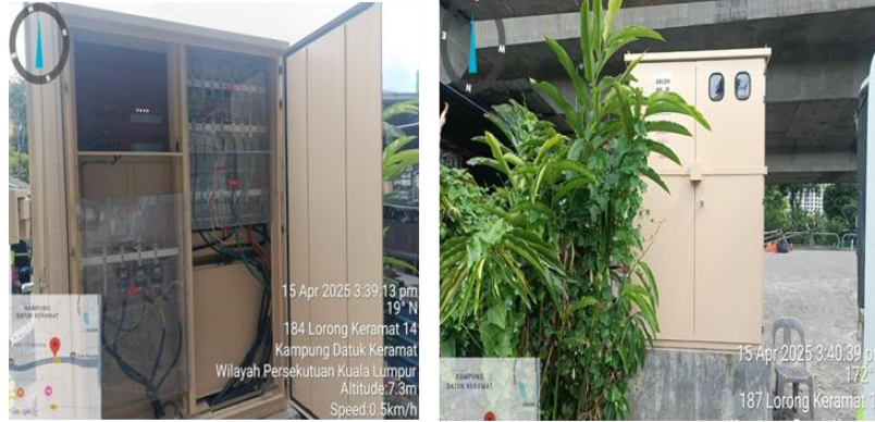
Replacement of Rusty Street Lighting Main Feeder Pillar
