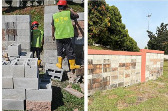
Installation of Noise Barrier
