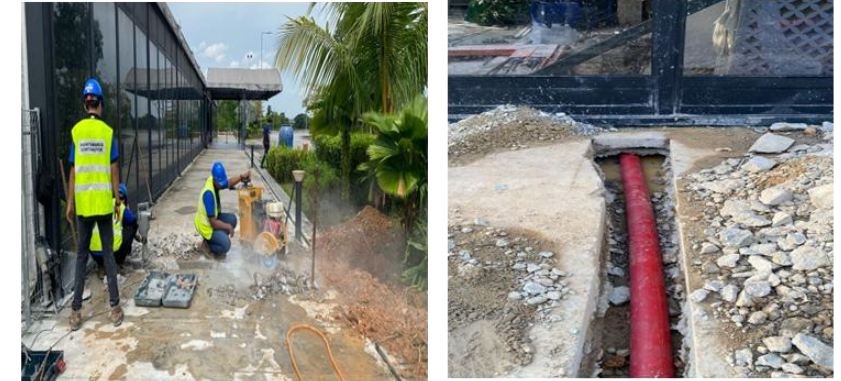
Upgrading of Power Cable for Air Conditioning
