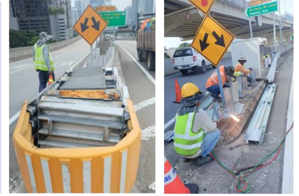
Replacement of Guardrails
