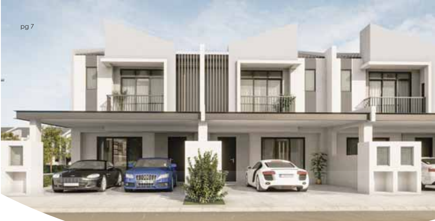
Bintang Bayu Sari - Double-Storey Terrace Homes
