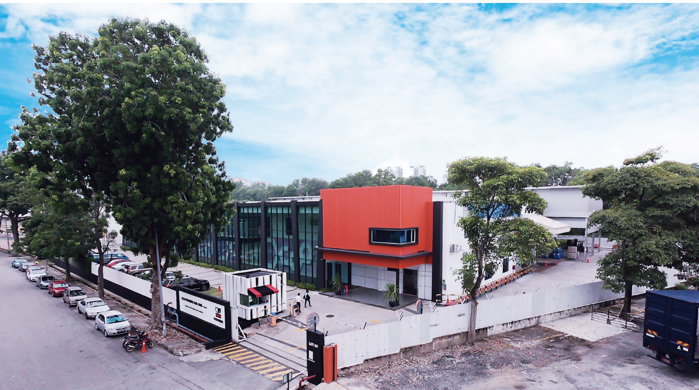
CCM Polymers new facility at Bangi
